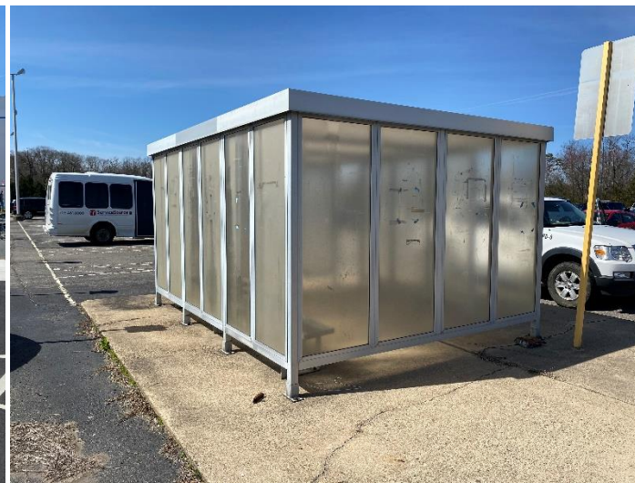
Existing Rte 208 PNR Lot Shelter
