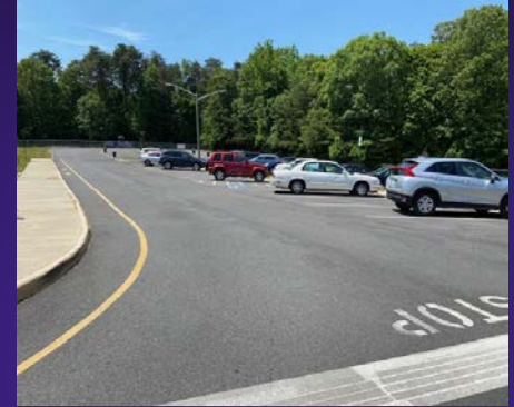
Parking Lot Improvements
